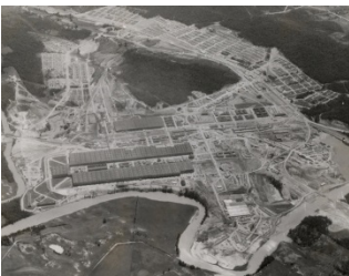
Aerial View Of K-25
