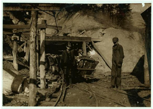
Greasers carried heavy buckets of grease that were used to lubricate gears on machinery and the wheels of coal cars. Couplers maneuvered the heavy coal cars into position and then connected them together. Injuries were common.
