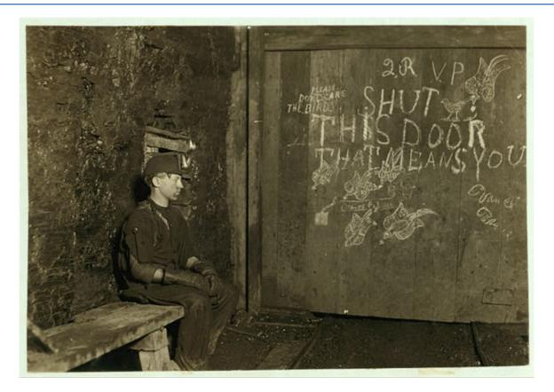
Ventilation was key to mine safety. Trappers or nippers open and closed doors along the mine tunnels. The doors had to remain closed to direct the flow of air into the side tunnels where the miners were working. The boys sat alone in the darkness for hours each day. It was so dark in the tunnel that Lewis Hine remarked that he had no idea there was writing on the door until the picture was developed. To stay awake, the boys whittled or trapped the rats that lived in the mine tunnels.
