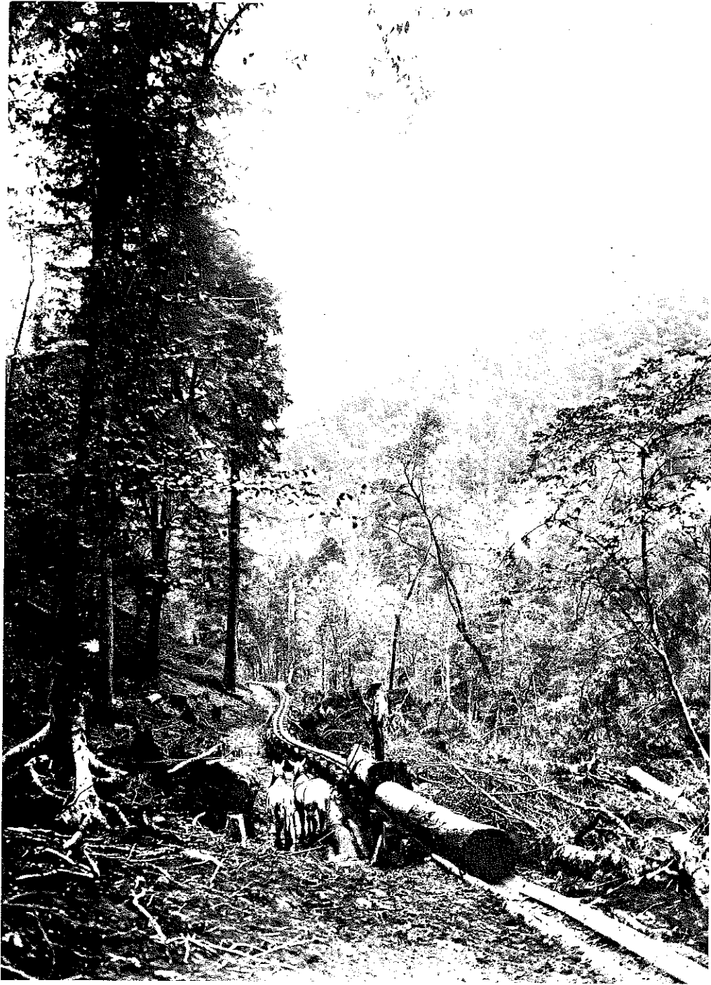
Flume Used to Transport Logs to Railroad. Collection of D. H. Tipton in National Park Headquarters, Gatlinburg.
